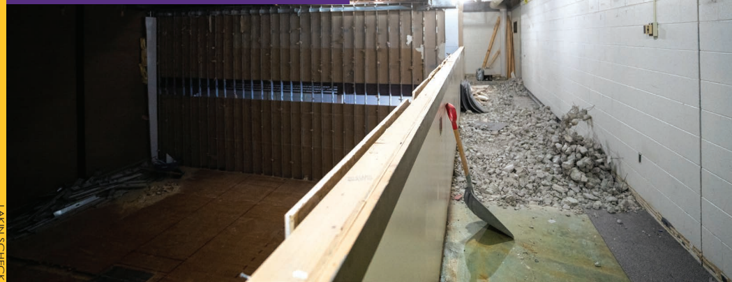
JUNE 7, 2023. Before removing the remaining cinder blocks for the new windows, workers add the edge pieces for the frames.
